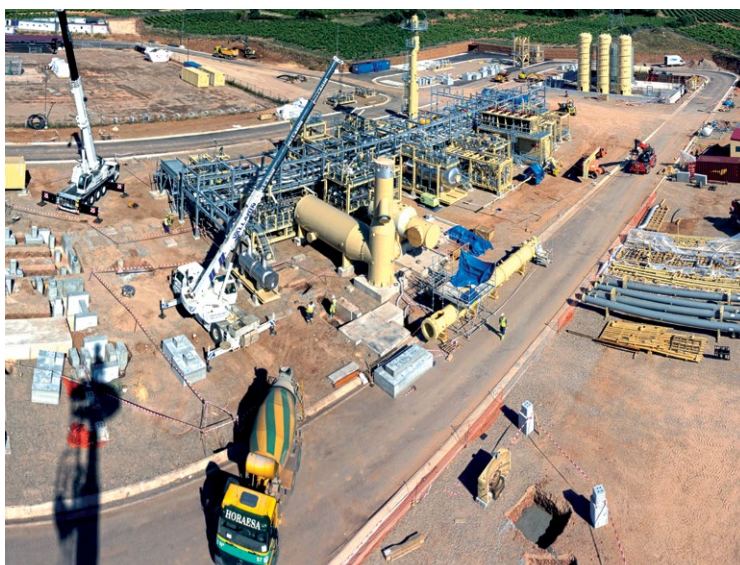
Process Plant Under Construction - Amine System
