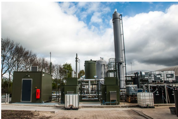
TEG Biogas Drying at Groot Zevent Vergisting
