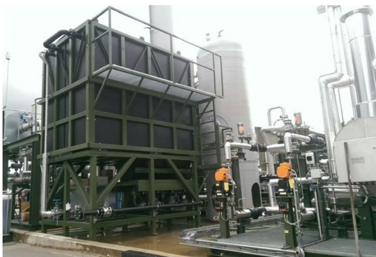
LAMINOL® installation Groot Zevert Vergisting
