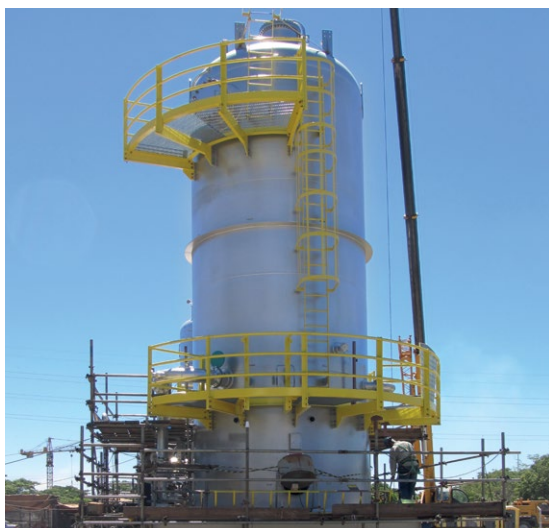
Compact Gas Flotation Skid
