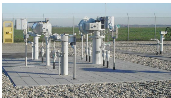
Gas Driven Double Acting Actuators Complete with Controls
